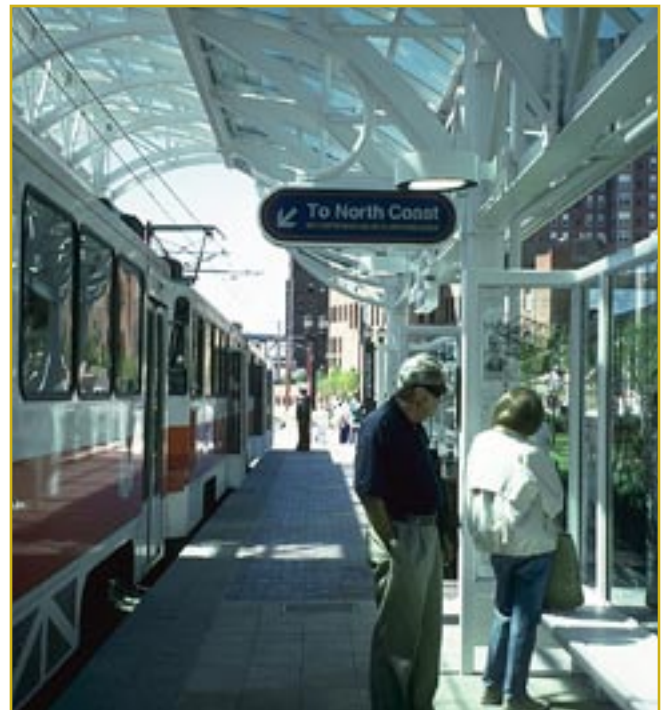
Light Rail Transit Station in Cleveland
