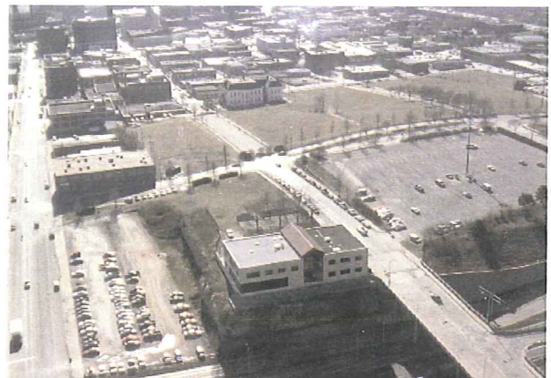
Performing Arts Center Site
